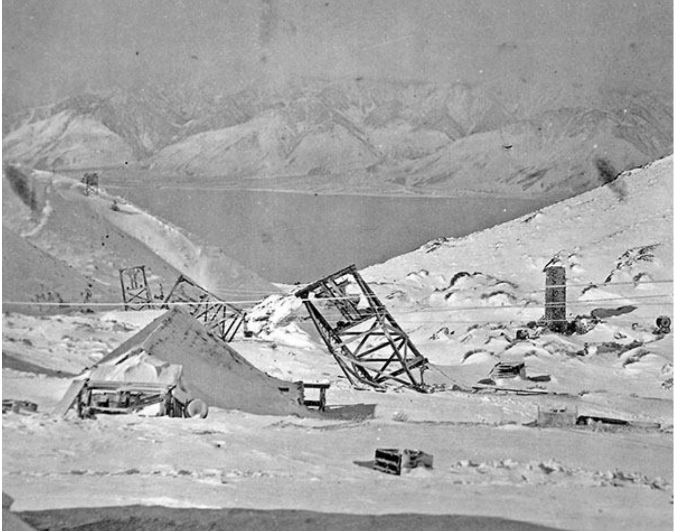
A snow storm knocks down tram towers and buries Cerro Gordo under a white blanket. (Photo L.D. Gordon Collection)
